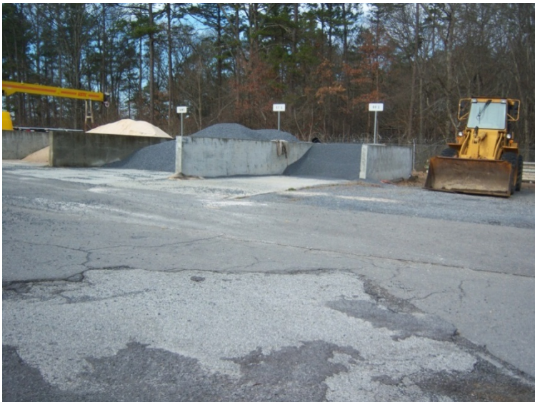
Photograph 3.2.8. Exterior graded aggregate stockpile bins at a Maintenance Headquarters.
