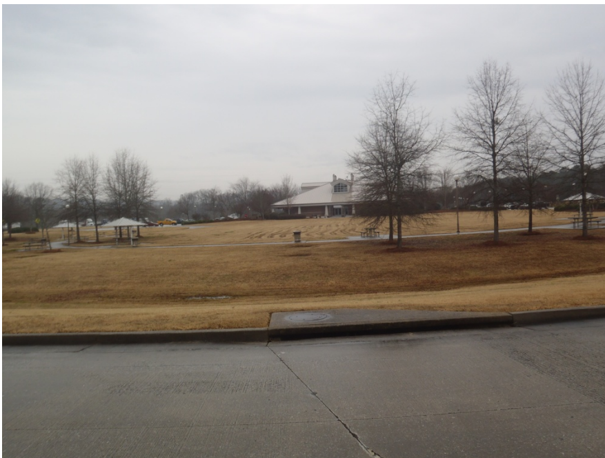
Photograph 3.3.2. A typical welcome center facility with building, sidewalks, picnic pavilions, trash receptacles, landscaping, roadway, and drainage features.
