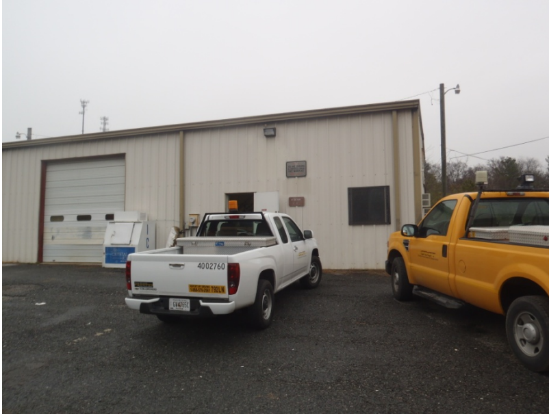
Photograph 3.2.7. A small Routine Maintenance Headquarters office, crew assembly area, and dry storage building.
