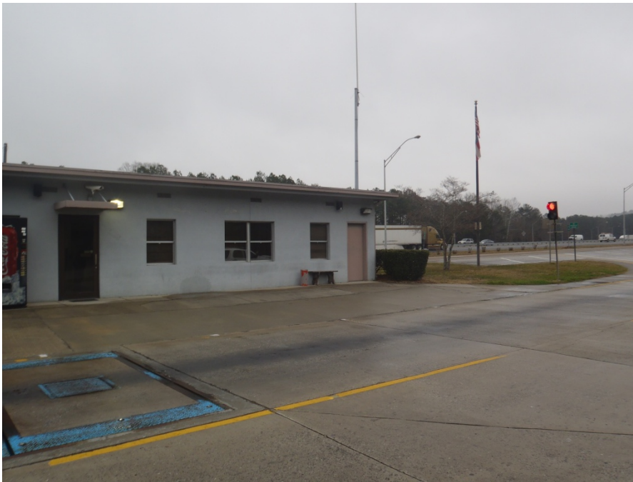
Photograph 3.4.3. A typical weigh station facility building with truck scales, landscaping, parking, and drainage features.
