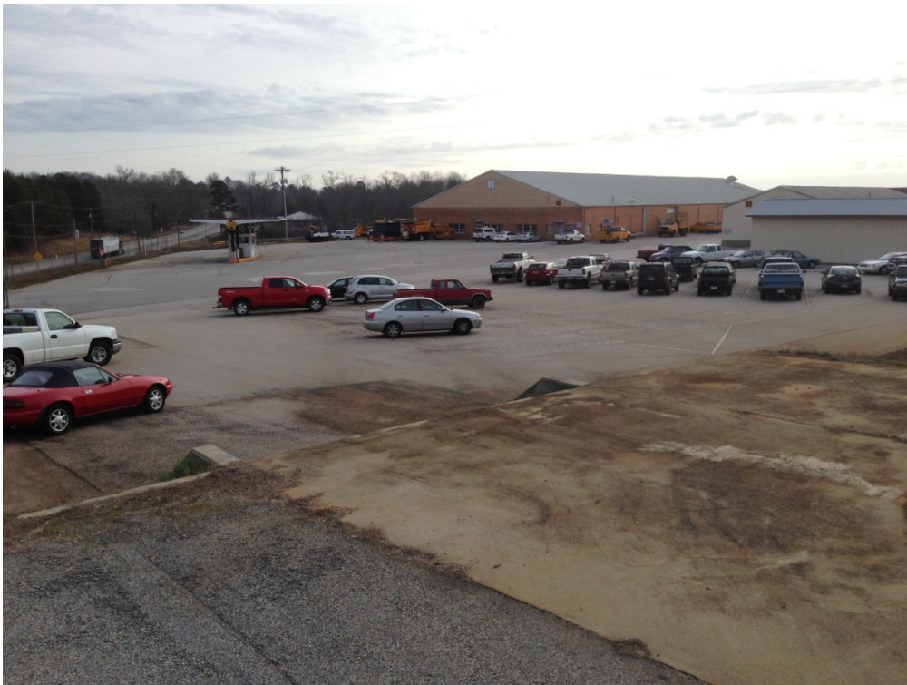
Photograph 3.2.1. A typical Maintenance and Storage complex, including Fueling Station, Maintenance Shop, Sign Shop, and exterior parking for GDOT vehicles and employee personal vehicles.
