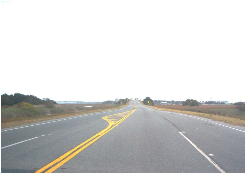
Photograph 3.4.2. A causeway across a coastal salt marsh with approach to bridge spanning a water body.
