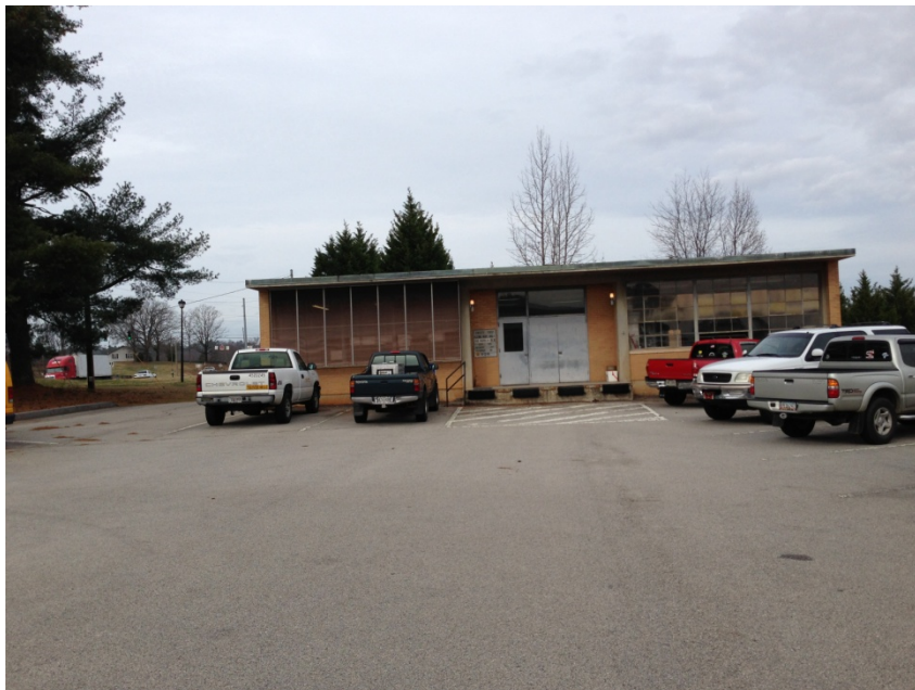
Photograph 3.1.3. A typical branch laboratory building with covered loading rack, parking, and modest landscaping.
