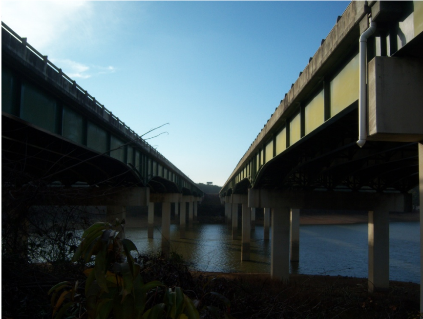
Photograph 3.4.5. Example of bridge over water body with deck drainage system.
