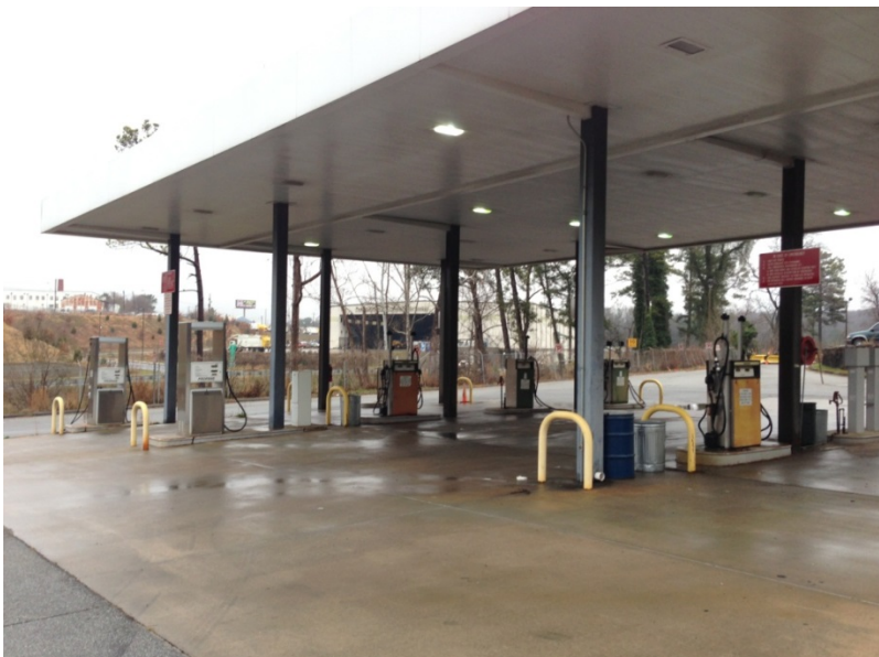
Photograph 3.2.12. A typical Fueling Station with canopy, concrete apron, and spill kits.
