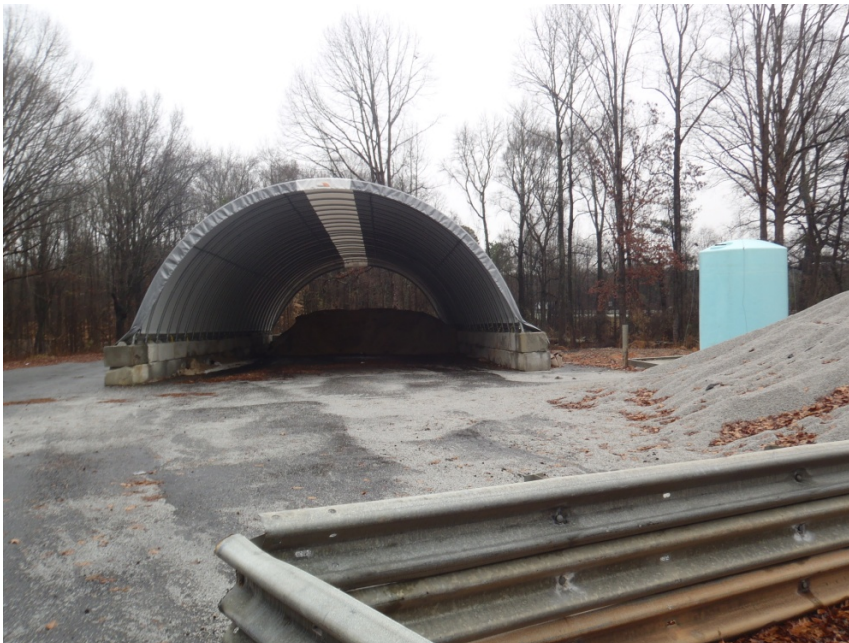
Photograph 3.2.14. A relatively new typical free-standing Salt Barn with brine solution tank and exterior aggregate stockpile at a stand-alone facility.
