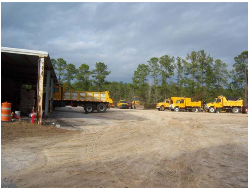
Photograph 3.2.6. A small Routine Maintenance Headquarters compound with unpaved vehicle and equipment parking.
