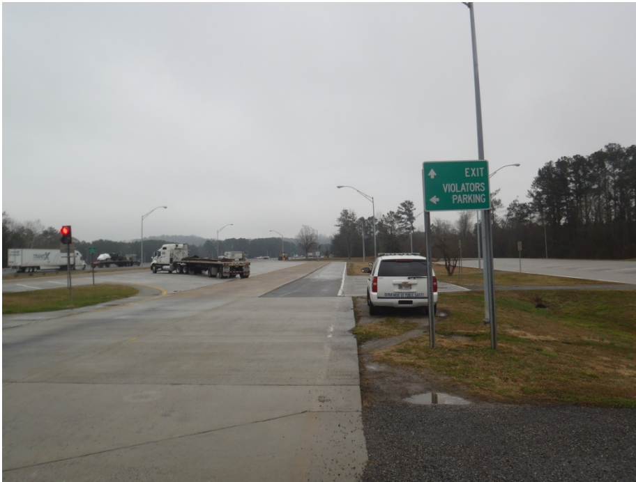
Photograph 3.4.4. Weigh station facility with parking area, landscaping, and drainage features.
